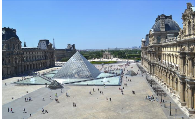
view of The Louvre entrance plaza from the 2 nd floor of the museum
